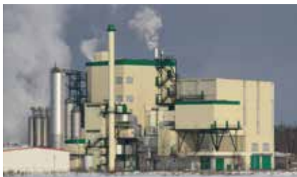
Hagenow/DE, 410°C, 34t/h, 46 barg
